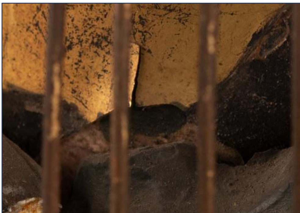
Figure 3-20: Lacquer Detaching from the Area Where the Large Branch of Br. 145 Was Previously Situated. Photograph: Author
